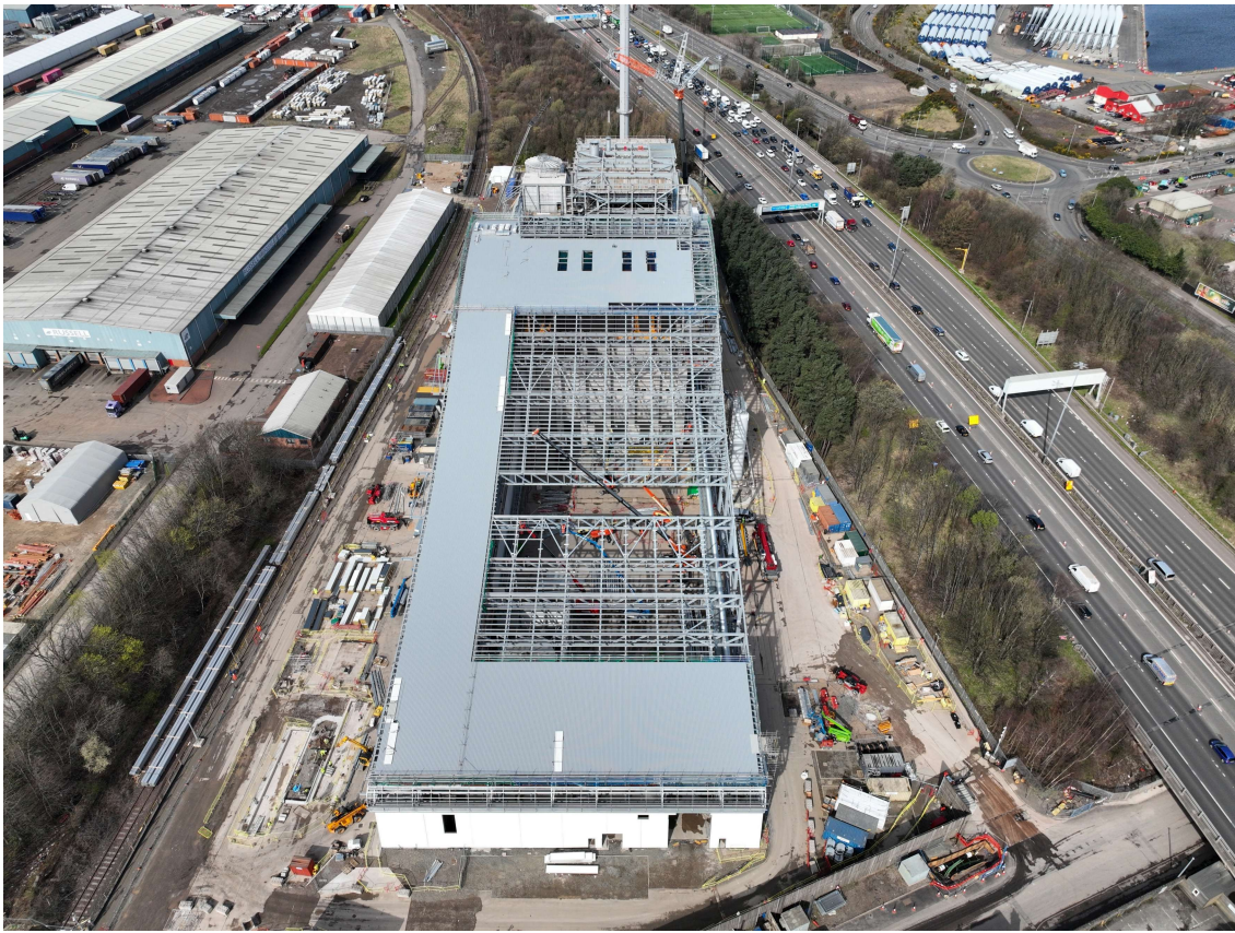
View of the South Clyde construction site
