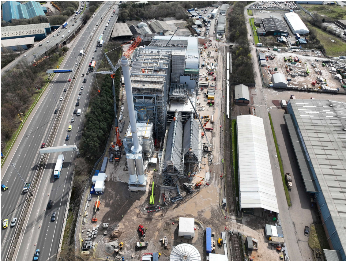
View of the South Clyde construction site
