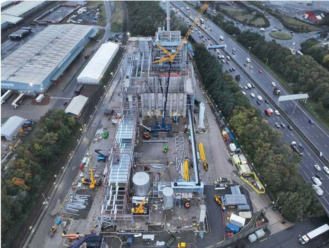
View of the South Clyde construction site
