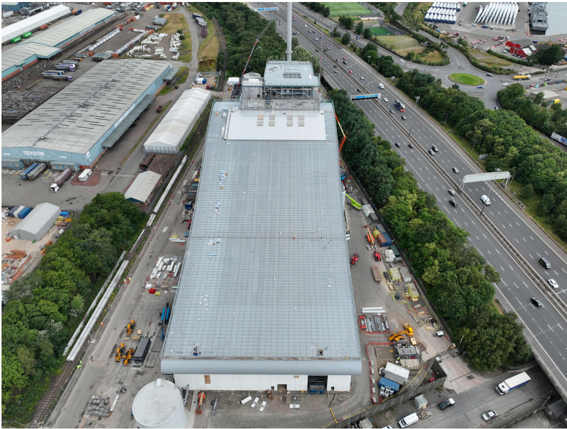
View of the South Clyde construction site
