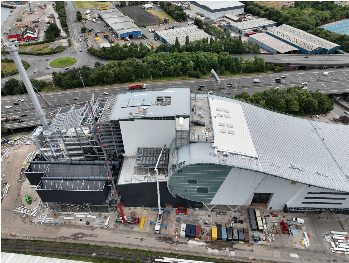
View of the South Clyde construction site
