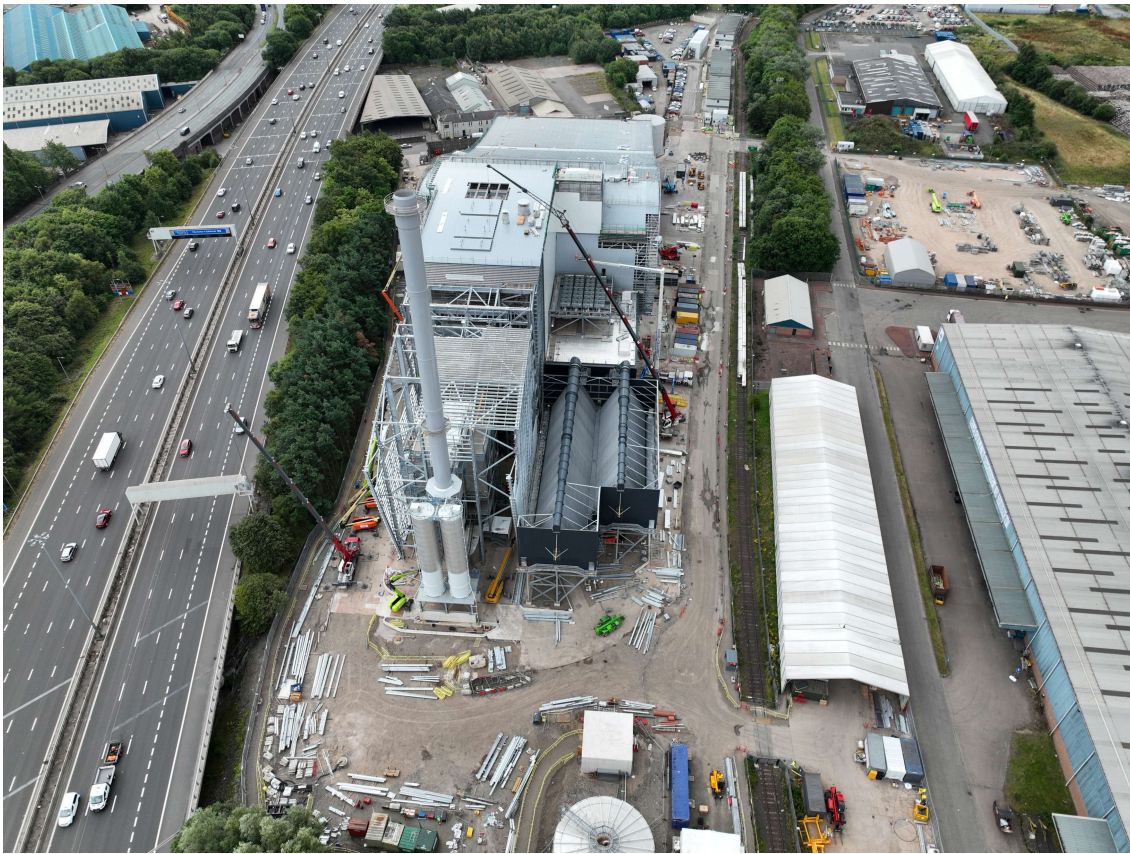
View of the South Clyde construction site
